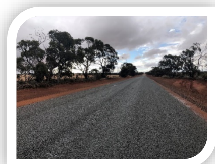
Figure 5: Morawa-Yalgoo sealing of road
