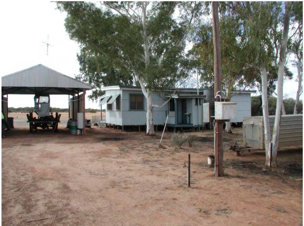
Morawa Gliding Club Infrastructure
